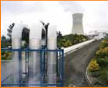
Cooling Towers, Ohaaki Geothermal Power Plant
